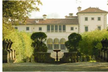
View of Main House from Casino Mound.
